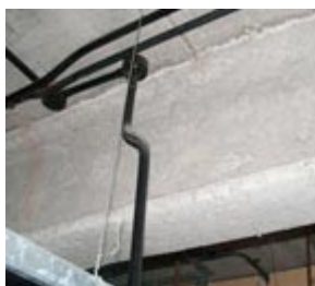
Typical example of sprayed asbestos to a steel beam
