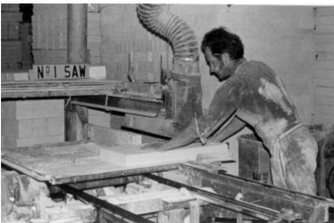
An operative working with Asbestos in 1970
