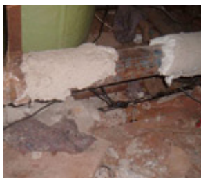
Asbestos lagging to heating pipes
