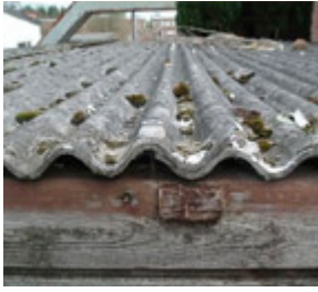
Corrugated asbestos cement sheeting to form roof coverings
