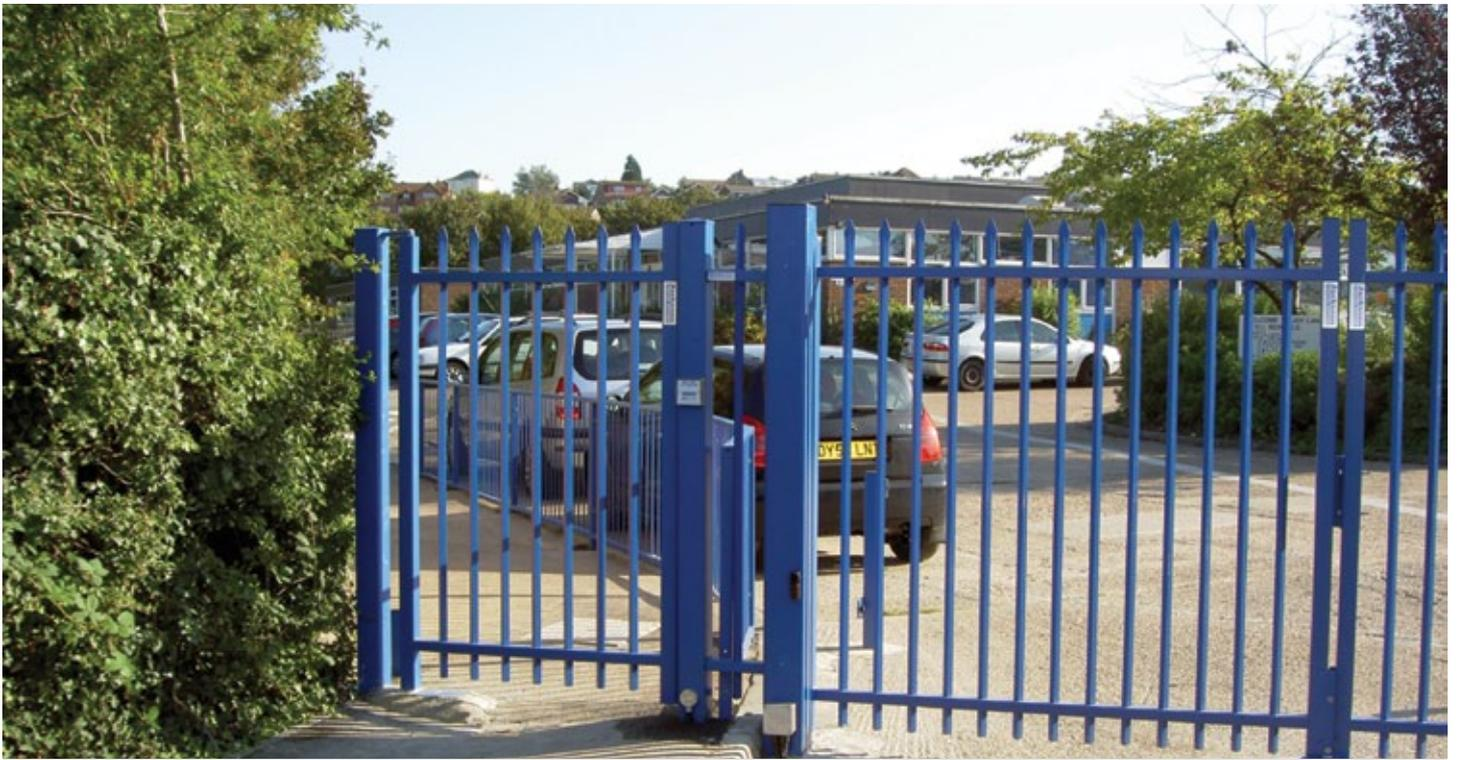
50.5.5 Posts should allow the construction of an unbroken panel to post chain and be of a non-brittle material
